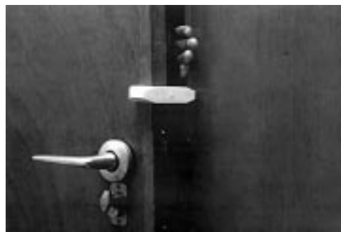
Figure 1 Rubber stopper in door at lock side preventing crushing of fingers.
